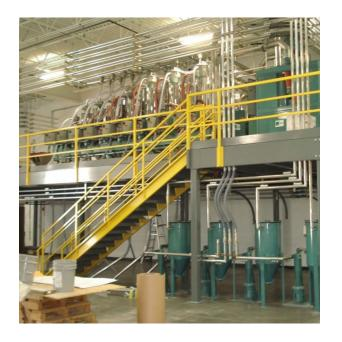
Air handling equipment for your facility, automated water treatment equipment for chemical processes, conveyors for materials handling and feed hoppers for automated equipment can all be easily moved to mezzanines. Easy access can be maintained to this equipment via the same mezzanine that supports it.
